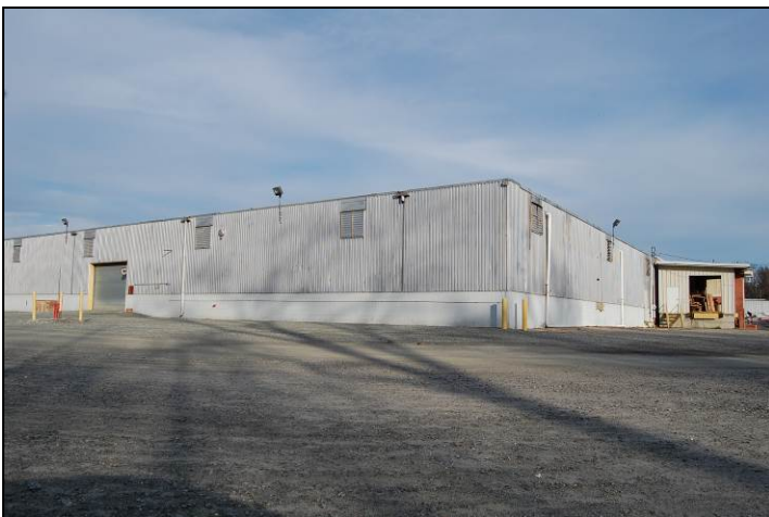
Figure 87. West side and south rear of c.1957-1965 addition at mill's southwest corner
