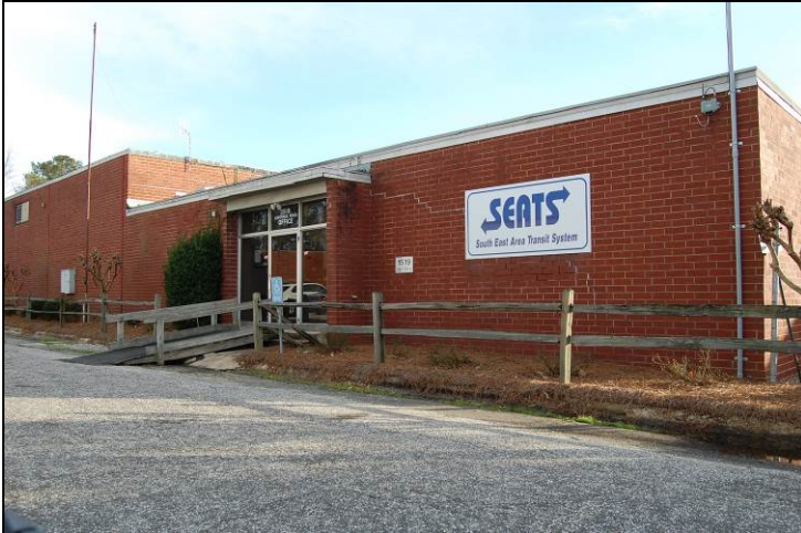
Figure 94. Looking at north-facing brick-veneered portion of concrete-block southeast addition from warehouse
