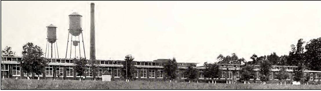
Figure 77. Jennings Cotton Mill, north front elevation with added water tower to rear, 1923 ( Southern Textile Bulletin , 1923:253)
