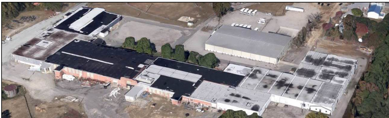
Figure 81. Modern Google Earth image of south rear of mill depicting boxy addition at southwest (far left corner), large roughly L-shaped wing with stained gray roofs at southeast (right), and freestanding warehouse to north (center right); note post-1957, on-ground water tank at far lower left
