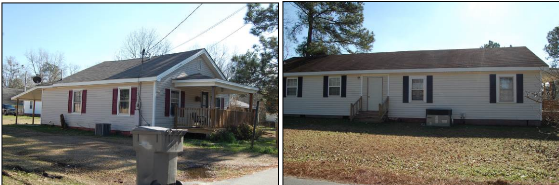
Figure 42. 68 Crescent St at left and 70 Crescent St (W. 24 th elevation) at right
