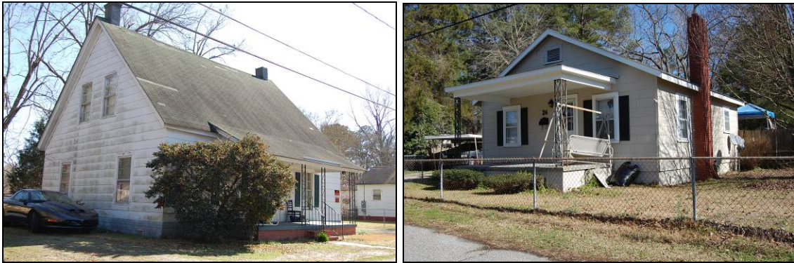
Figure 21. 22 Albion St at left and 24 Albion St at right
