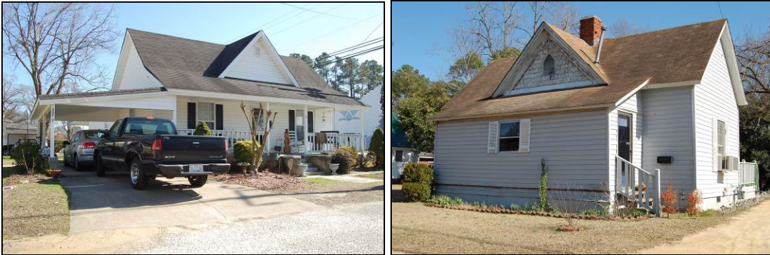
Figure 17. 6 Albion St at left and 8 Albion St at right
