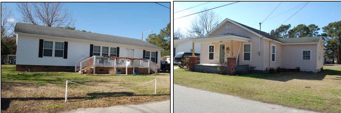
Figure 36. 32 Bradford St at left and 30 Bradford St at right
