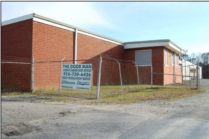
Figure 86. West-facing elevation of 1927 knitting room with windows hidden by later brick veneer
