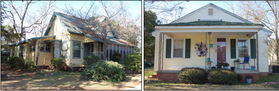
Figure 25. 19 Albion St at left and 21 Albion St at right
