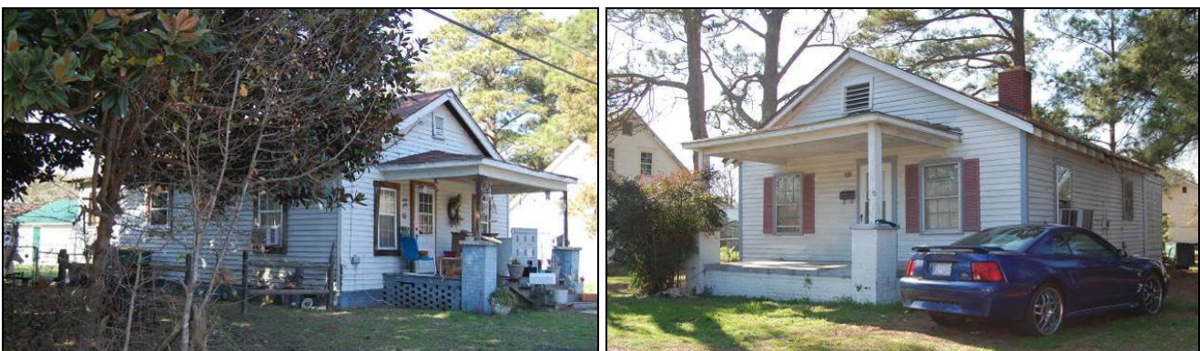
Figure 14. Largely intact Type B houses at 65 Crescent Street, at left, and 69 Crescent, at right
