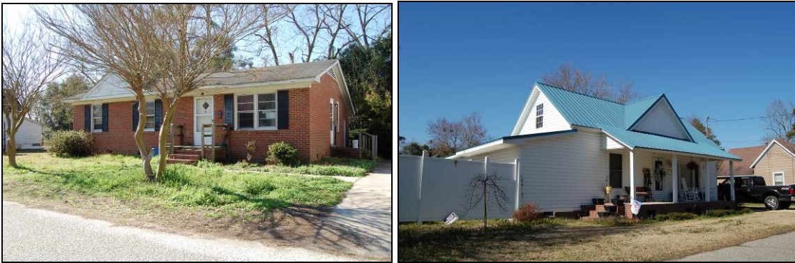
Figure 23. 11 Albion St at left and 13 Albion St at right
