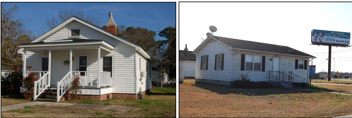
Figure 63. 103 Elba St at left and 1205 W 24 th St [Lot 121] at right
