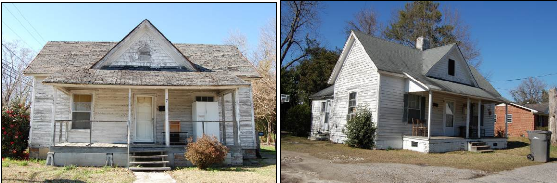
Figure 22. 7 Albion St at left and 9 Albion St at right
