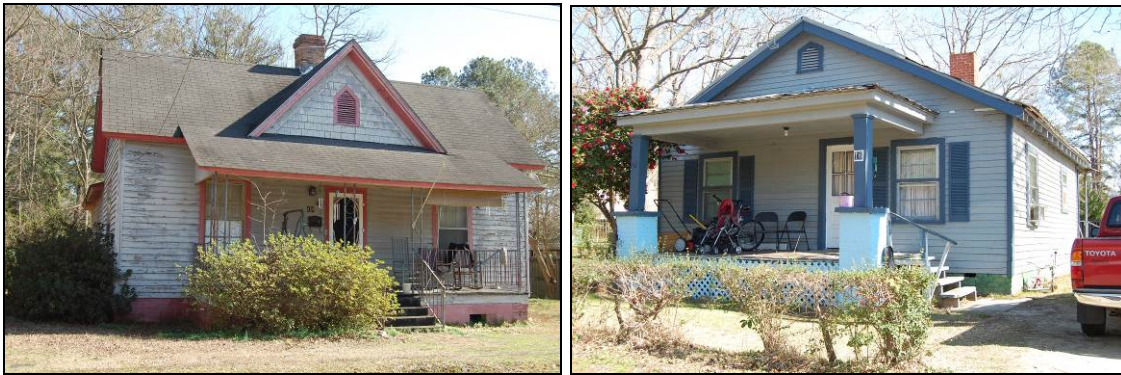
Figure 19. 14 Albion St at left and 16 Albion St at right
