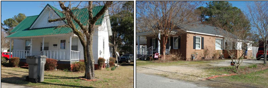
Figure 18. 10 Albion St at left and 12 Albion St at right
