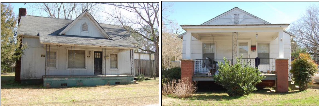
Figure 20. 18 Albion St at left and 20 Albion St at right
