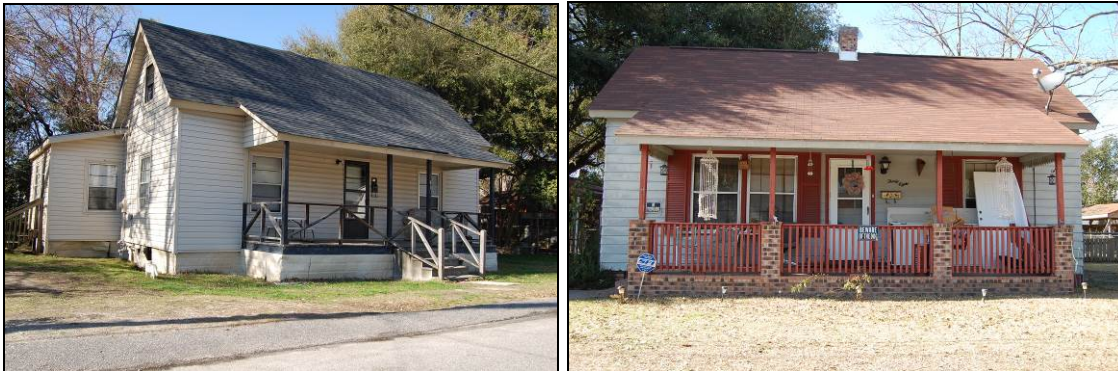
Figure 34. 40 Bradford St at left and 38 Bradford St at right
