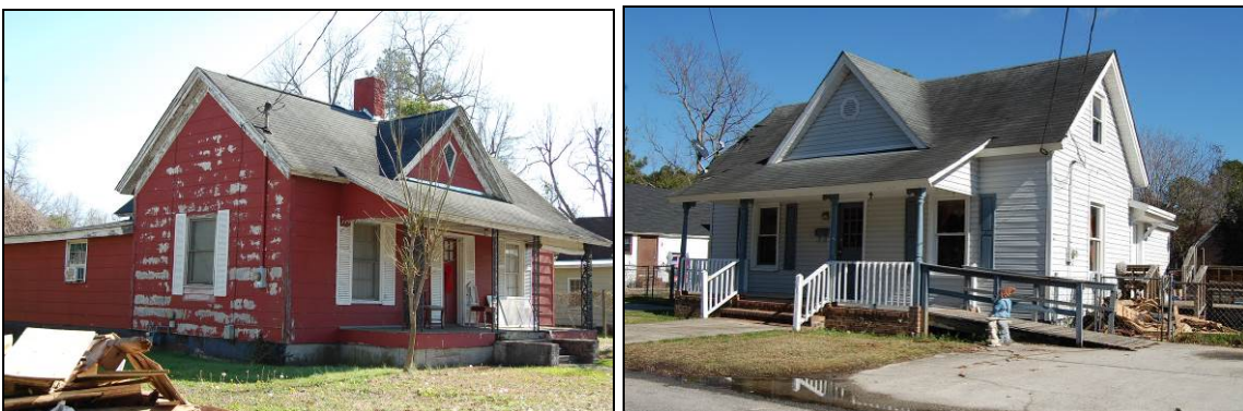
Figure 28. 43 Bradford St at left and 41 Bradford St at right
